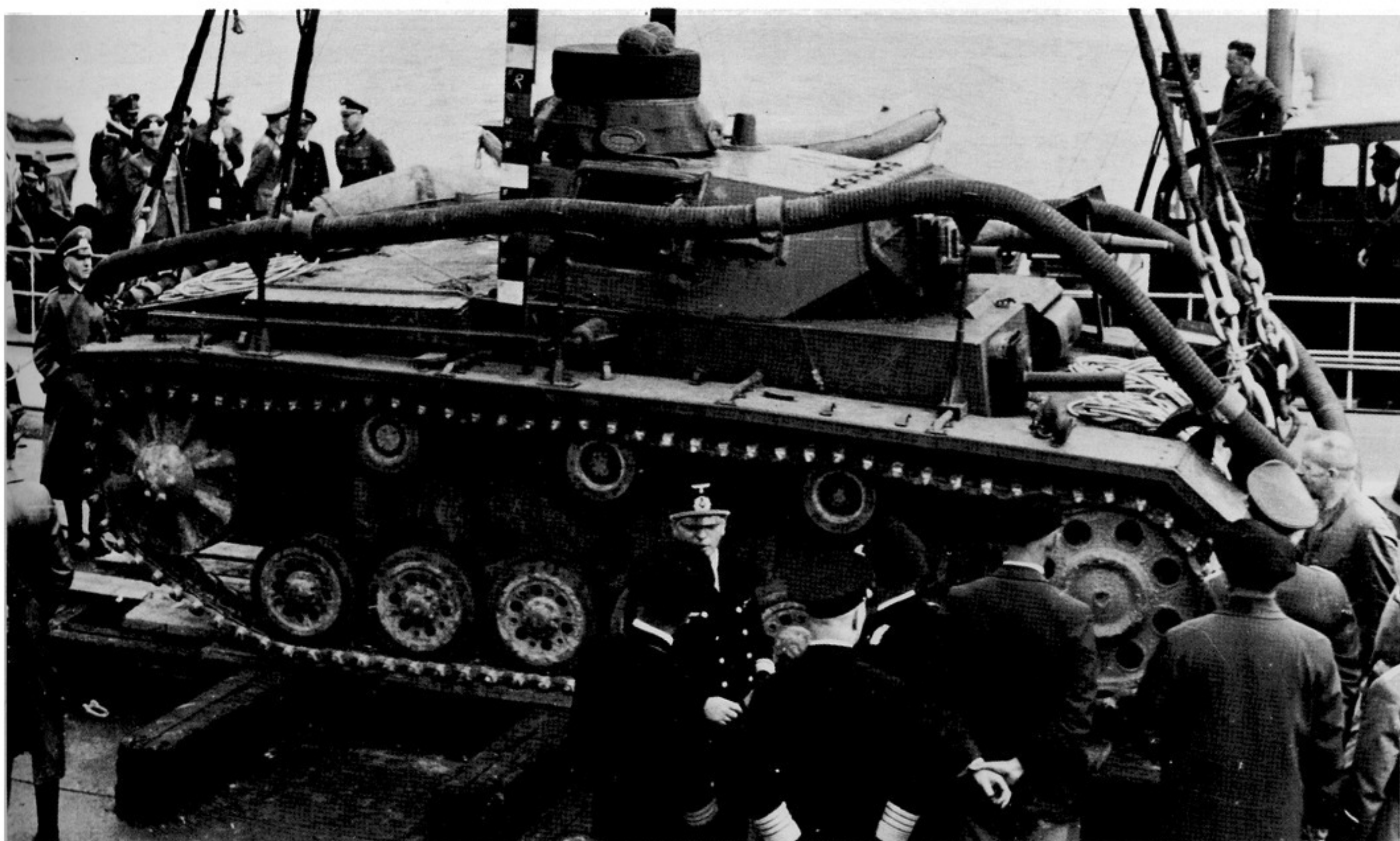
For Operation "Sealion", the invasion of England, Panzer III and IV were prepared for underwater action. This picture shows a Panzer III Ausf. F with closed openings and an air hose for the engine and the fighting compartment.
